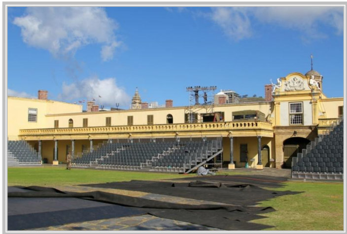
Photo 1: The black rubber mats that were laid down to protect the old paving stones were all lifted up by the strong southeaster wind despite being very heavy
